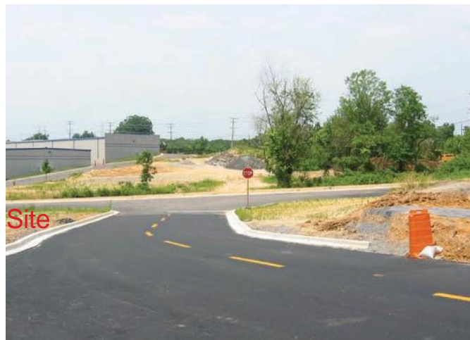
Valley Stream Avenue after paving
