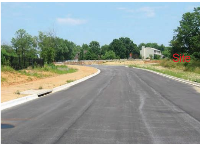
Dino Drive after paving
