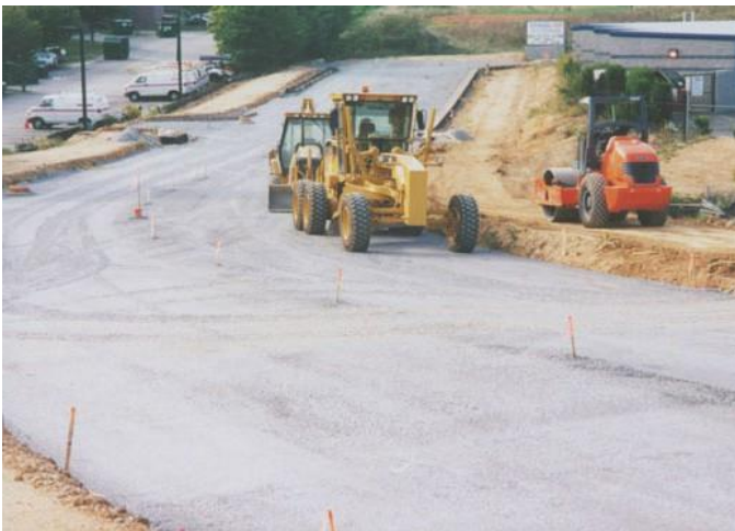
Dino Drive - under construction
