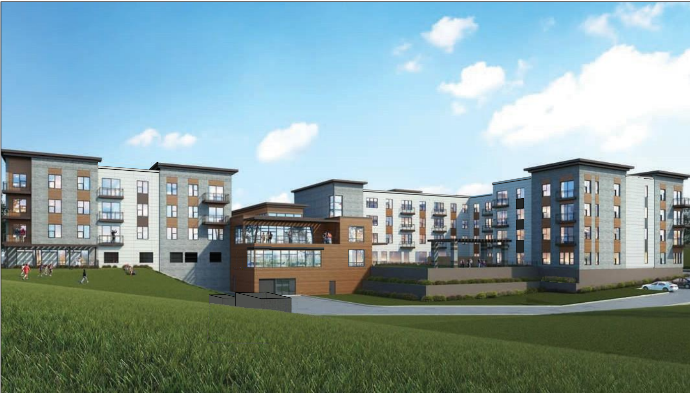
View from Rear of Facility
