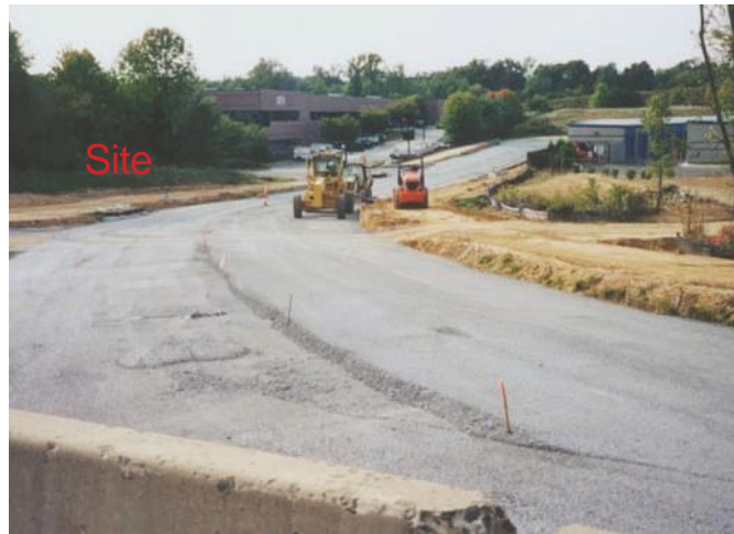
Dino Drive - under construction
